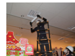
Installation of LED lighting
